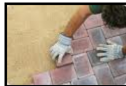
A worker paving the driveway
